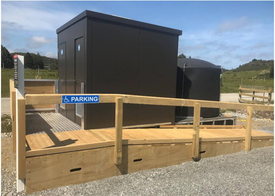
New toilet block at Kokatahi.
